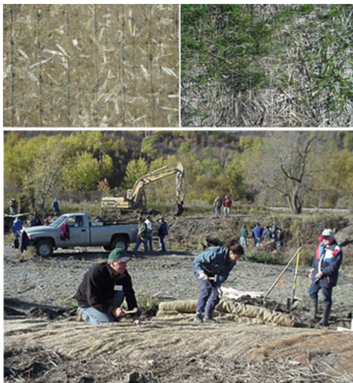
Fig. 32. Hemp-based erosion control blanket. Top left: Close-up of 100% hemp fiber blanket. Top right: Grass growing through blanket. Bottom: Demonstration of installation of blanket, near La Rivière, Manitoba. (Courtesy of Mark Myrowich, ErosionControlBlanket.com)
