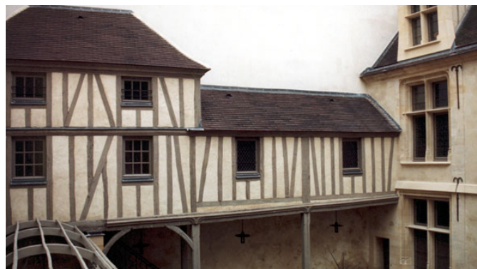
Fig. 26. Renovation of plaster walls of a traditional timber frame 16 th century house (Mansion Raoul de la Faye, Paris) with Isochanvre® lime-hemp conglomerate. (Courtesy of M. Périer, Chènovotte Habitat, France.)
