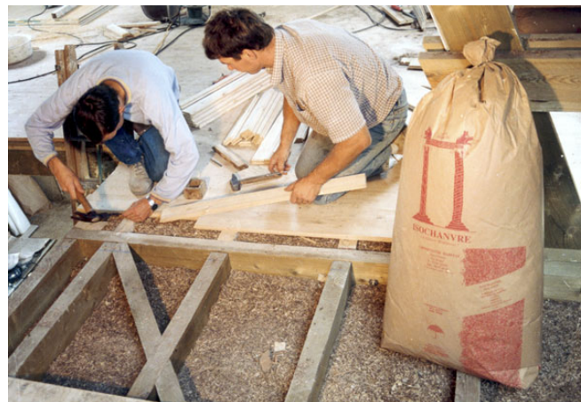
Fig. 21. Loose Isochanvre® thermal insulation being placed between joists. (Courtesy of M. Périer, Chènovotte Habitat, France.)
